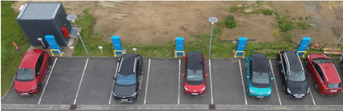
Figure 3: Aerial photo of the finished MADELAINE demonstrator; the power converters and adaptive DC switch matrix are located in the grey container on the top left of the photo, the charge points 1 - 10 are located in the blue cabinets
